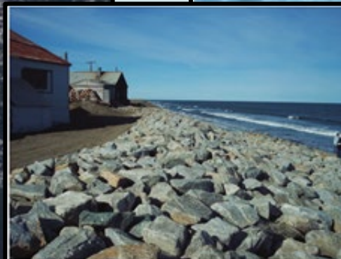
Figure 3-3. A revetment designed by the U.S. Army Corps of Engineers protects a street and buildings at Shishmaref in northwestern Alaska. Mikal Hendee photo.
