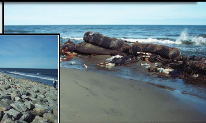
Figure 3-3. A revetment designed by the U.S. Army Corps of Engineers protects a street and buildings at Shishmaref in northwestern Alaska. Mikal Hendee photo.
