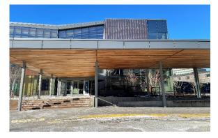
**Flashing:** Metal flashing (edging) torn off from the canopy at the APK front entrance during the blizzard in November 2023 was pieced back together and replaced in March 2024.
